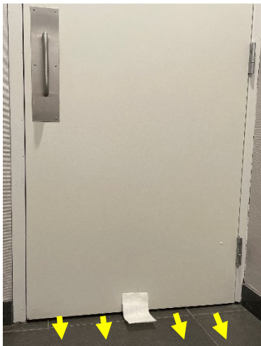
Figure 7. View from inside a negative pressure room.
