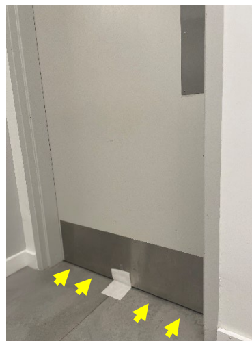
Figure 8. View from inside a positive pressure room.
