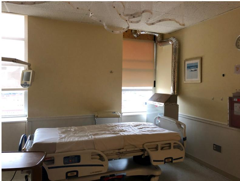
**Photo 1:** Temporary AIIR negative isolation room. Air is exhausted
