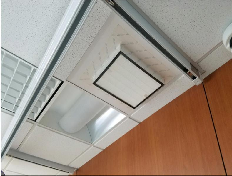
**Photo 2:** Installation of HEPA filter on return air diffuser in order to create temporary neutral/negative pressure for single patient room.
