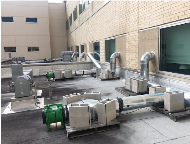
**Photo 3:** Single patient room negative air configuration through exterior windows. Air is exhausted by HEPA filtered air at roof level.
