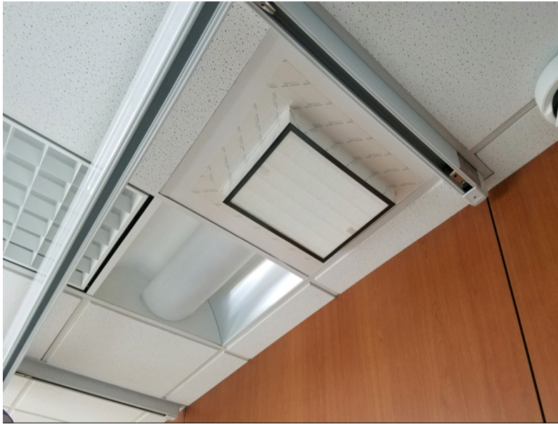
Photo 2: Installation of HEPA filter on return air diffuser in order to create temporary neutral/negative pressure for single patient room. Photo Courtesy of Naval Hospital Camp Pendleton, Camp Pendleton, California
