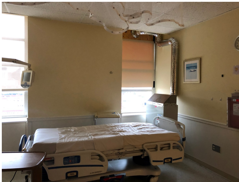
Photo 1: Temporary AIIR negative isolation room. Air is exhausted by HEPA filtered air outside.
